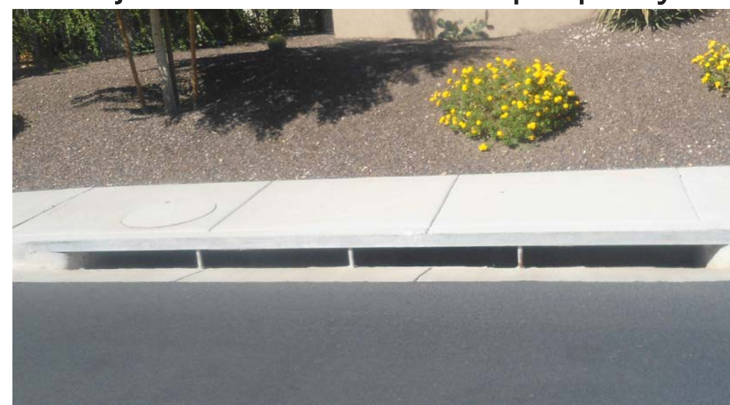
Figure 1: Storm drain system adjacent to residential property.
