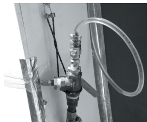
Fig 9 (Bottom Left): Control Valve for the water supply to the misters.
