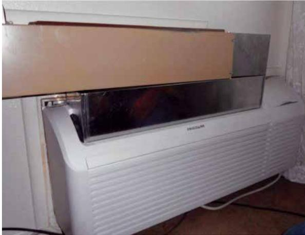
The Frigidaire PTAC units are controlled by a simple, non-programmable thermostat on the living room wall near the door to the bedroom, at the approximate center of the unit.
