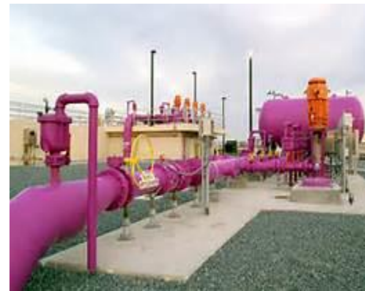
Purple Pipe (Secondary plumbing to deliver a separate water supply for non-potable use)
